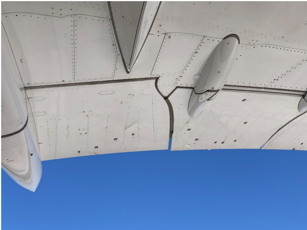
Picture 5: aircraft damage.
