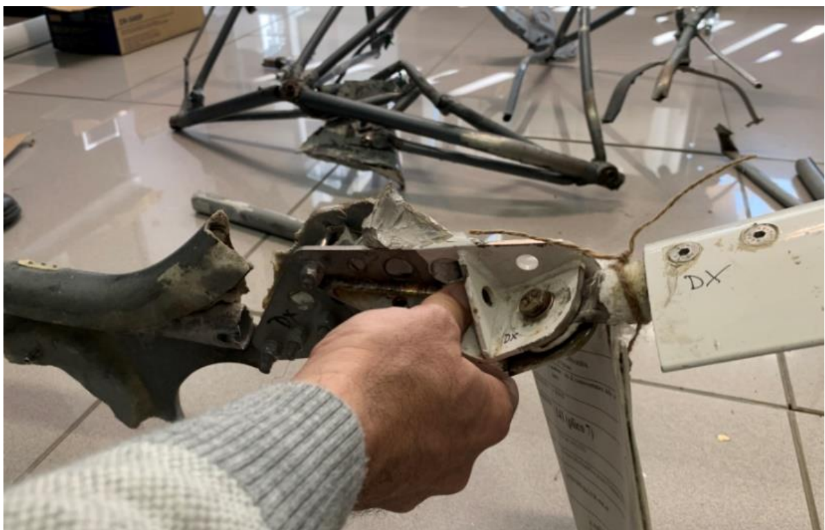
Photo 14: internal rib wing strut fixing point right side and wing strut fixing plate right side.
