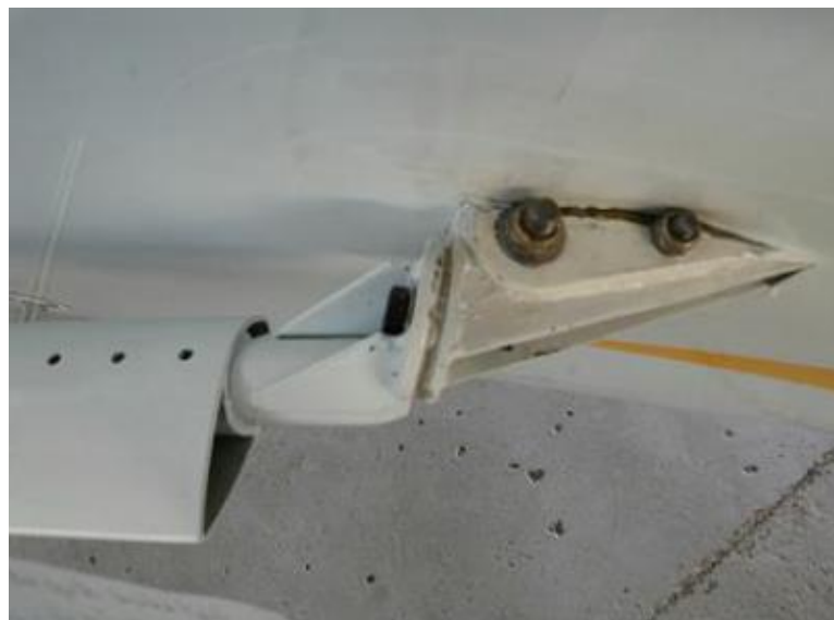
Photo 2: upper fixing point of the wing strut to the lower part of the wing (right wing).
