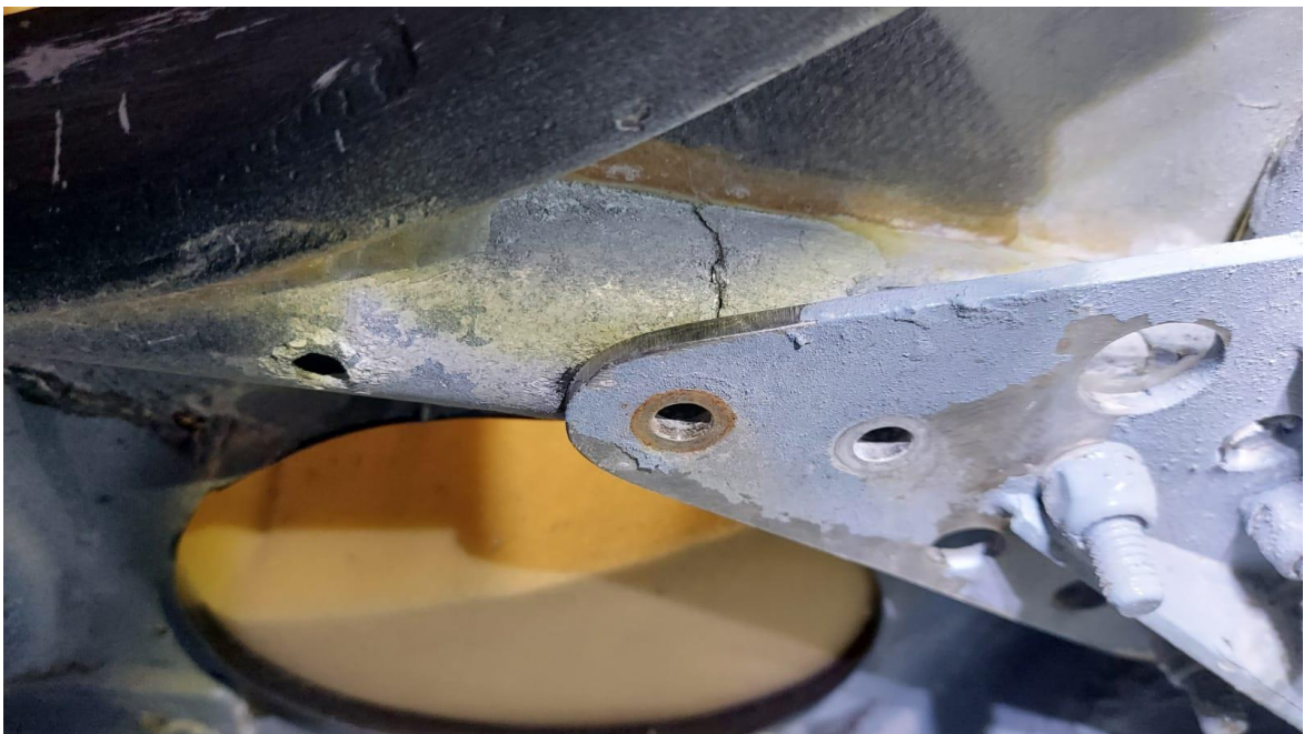
Photo 24: fracture of the aluminium tubular of the rib at the bolt securing the wing strut fixing plates, found on an Italian Seamax M-22 aircraft after the accident at I-7608.
